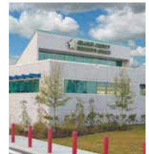
Orange County Sheriff's Office Building Sector II
